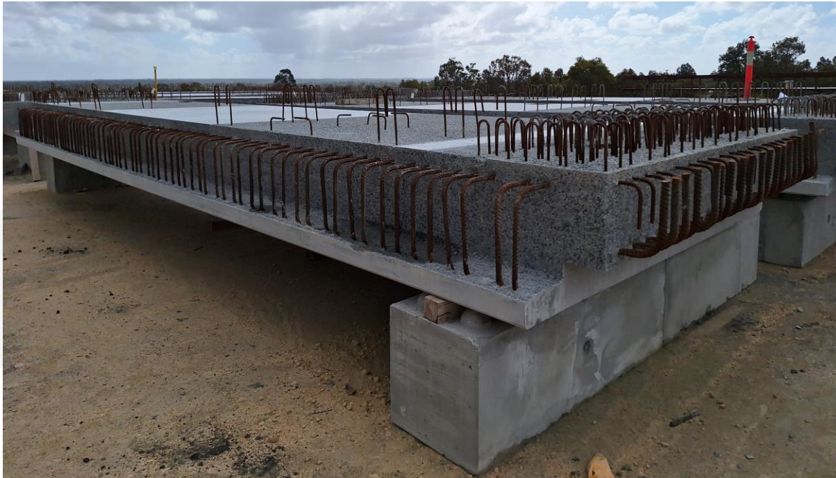
Metronet WA Project Byford Rail Extension – Viaduct Concrete Planks
