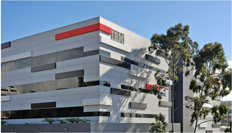
Fugro Building West Perth, WA
