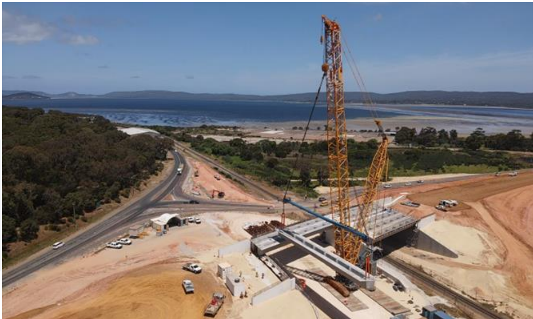
Albany Ring Road Project under construction 2023
