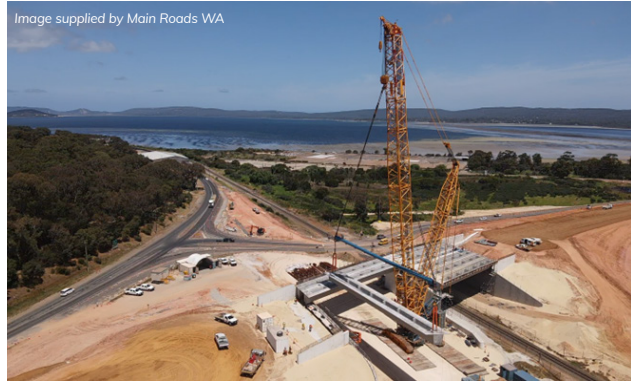
Installation of beams for Bridge 1871 of the Albany Ring Road
