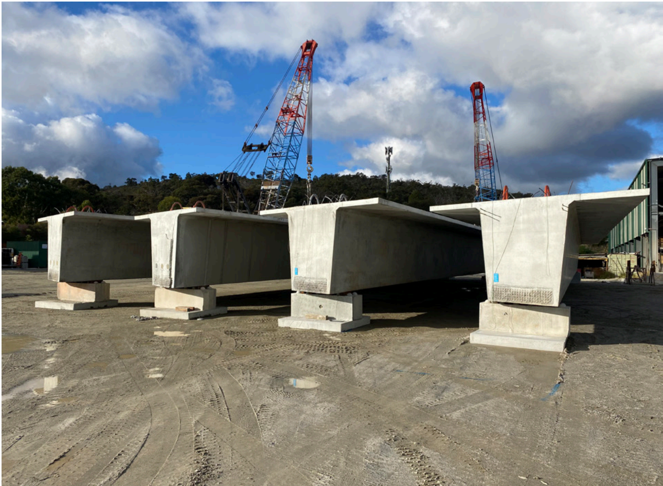
Albany Ring Road Bridge Beams
